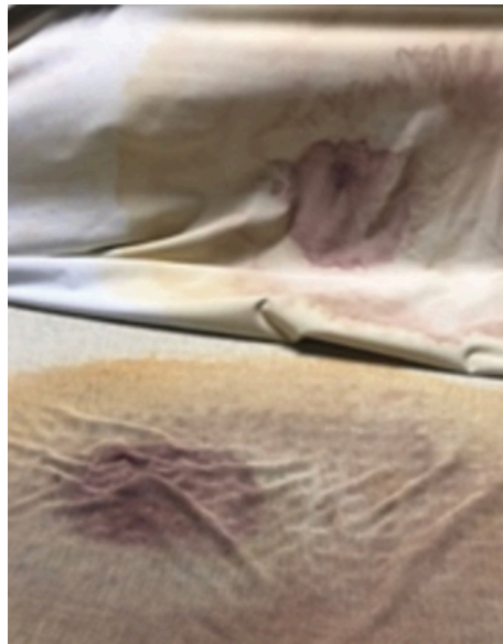
Image 2: Staining on bottom of integrated mattress cover and top of fire barrier
